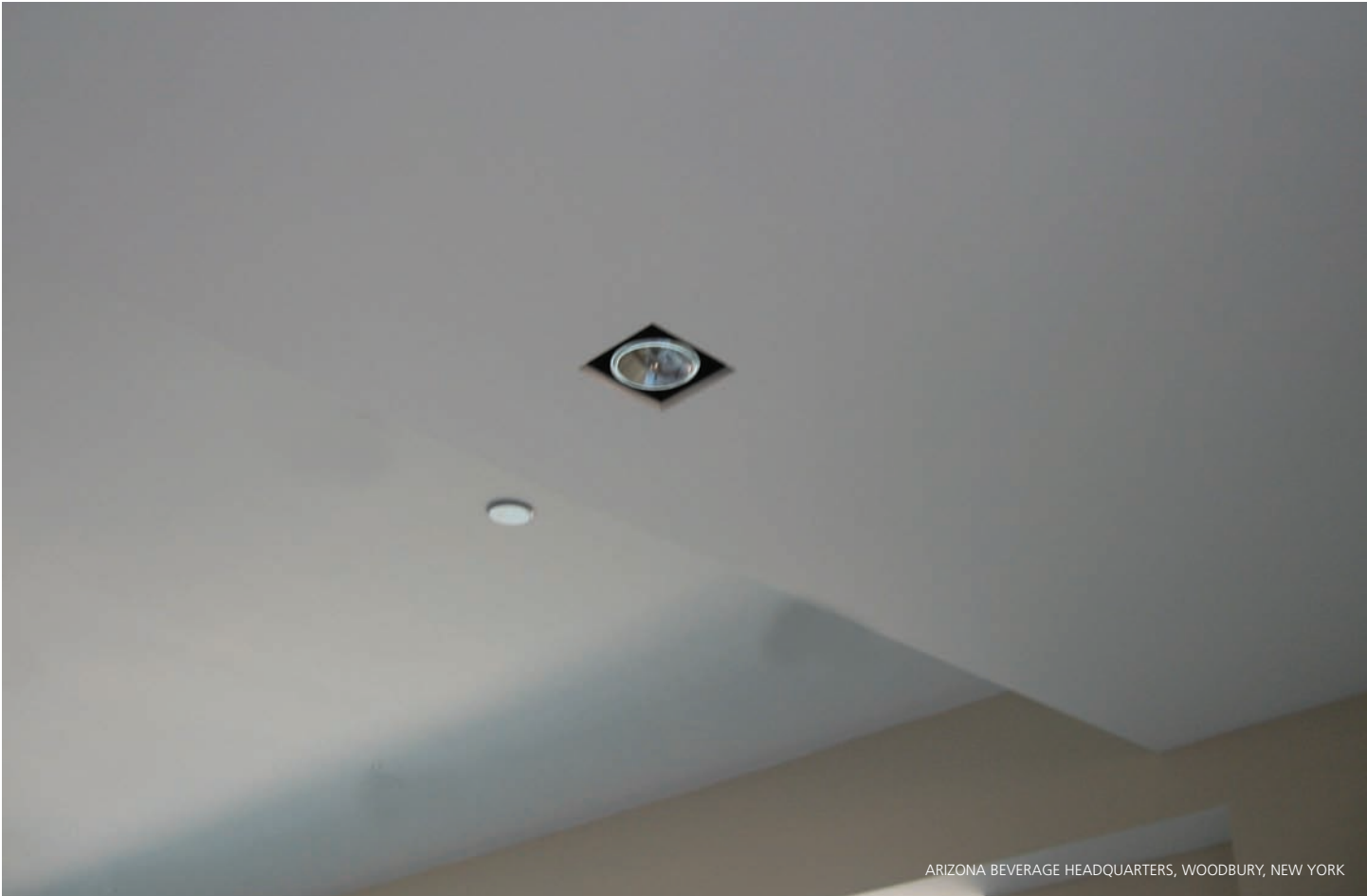
ARIZONA BEVERAGE HEADQUARTERS, WOODBURY, NEW YORK
