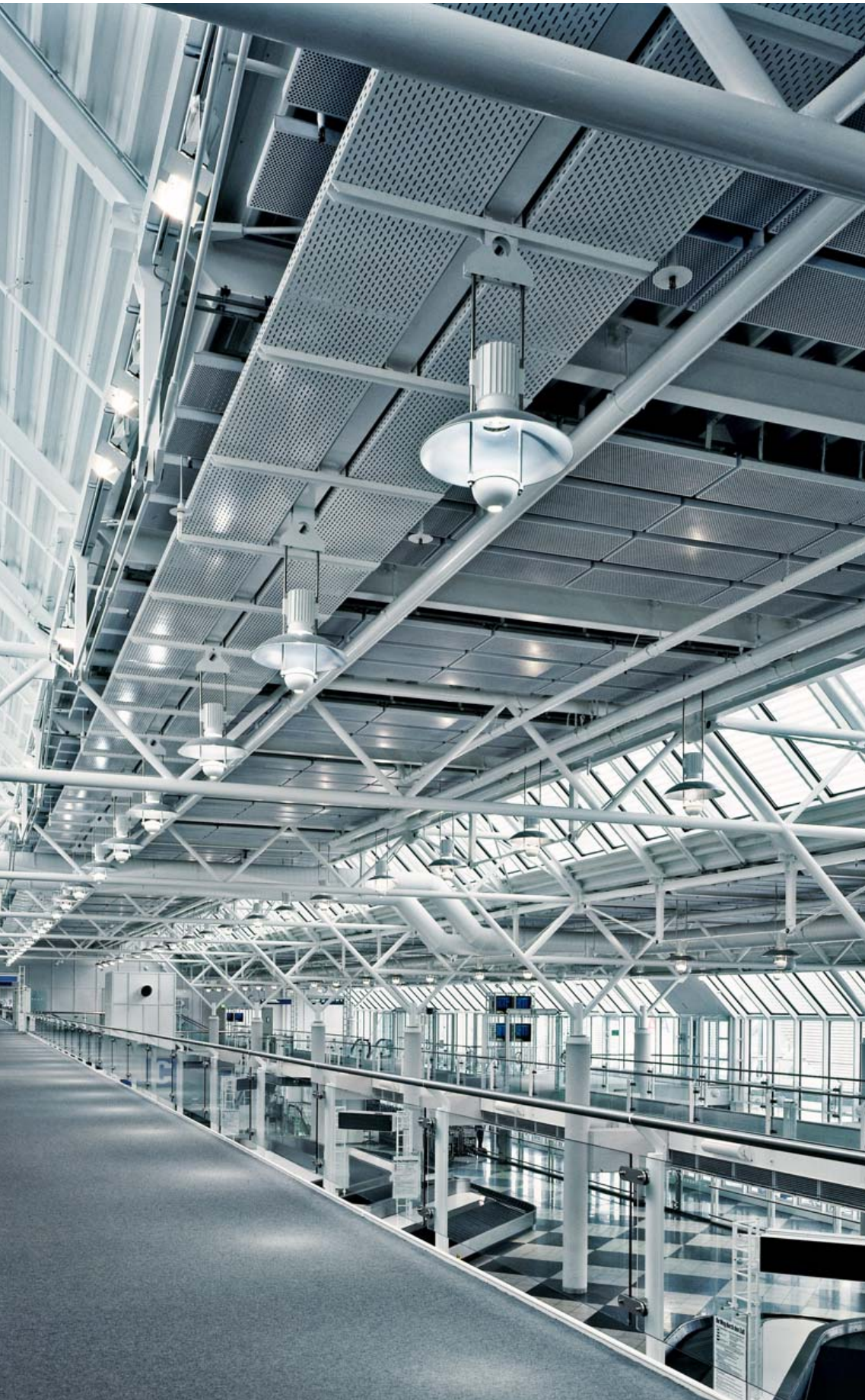
Airport. Munich Airport, Munich, Germany. Photo: Udo Kowalski.
